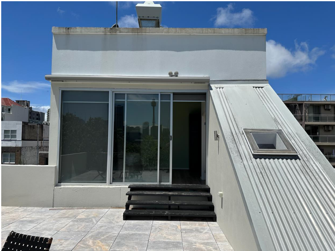
Figure 11: View of Unit 15 viewed from rooftop terrace.
