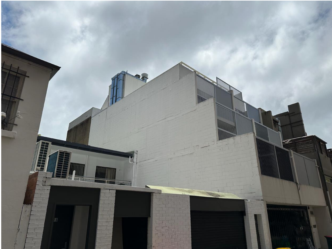
Figure 6: Southern elevation viewed from Earl Street, facing north west.
