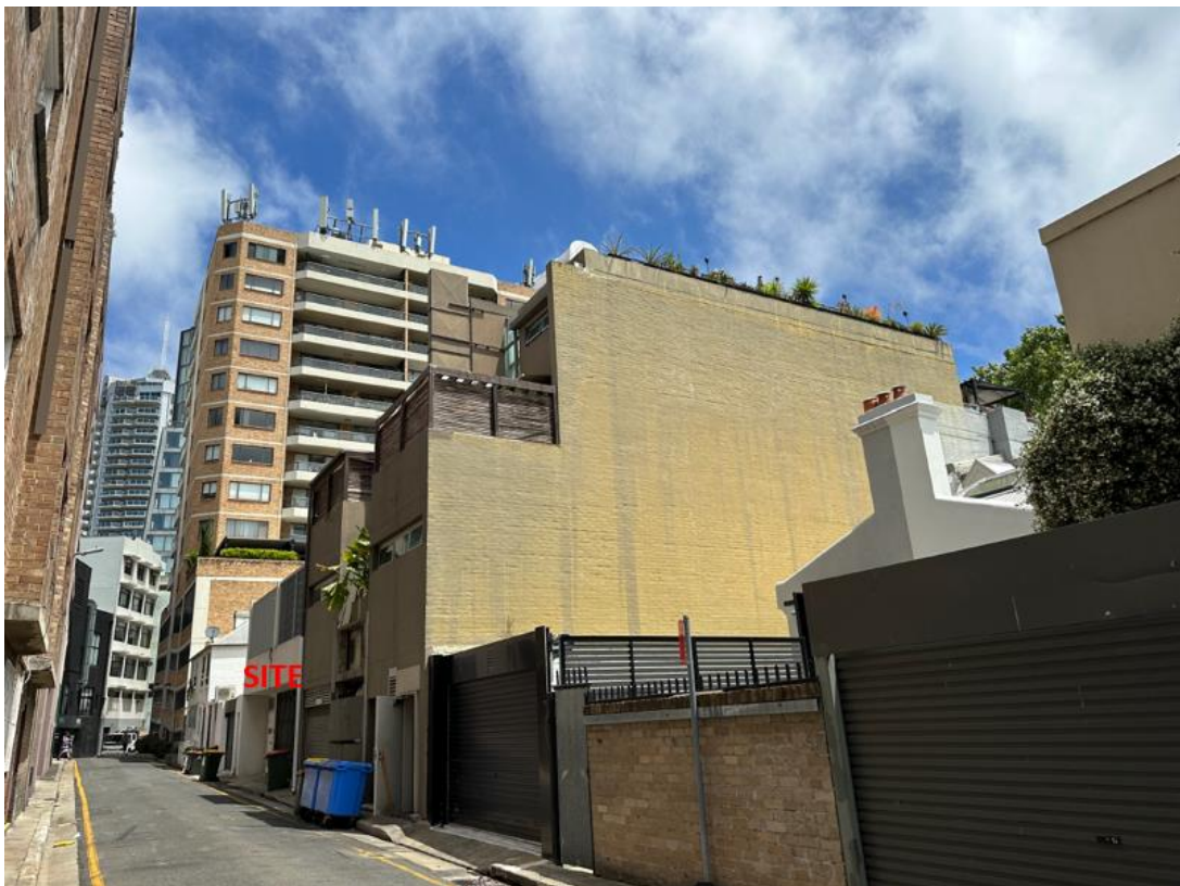
Figure 7: Site viewed from Earl Street, facing south.
