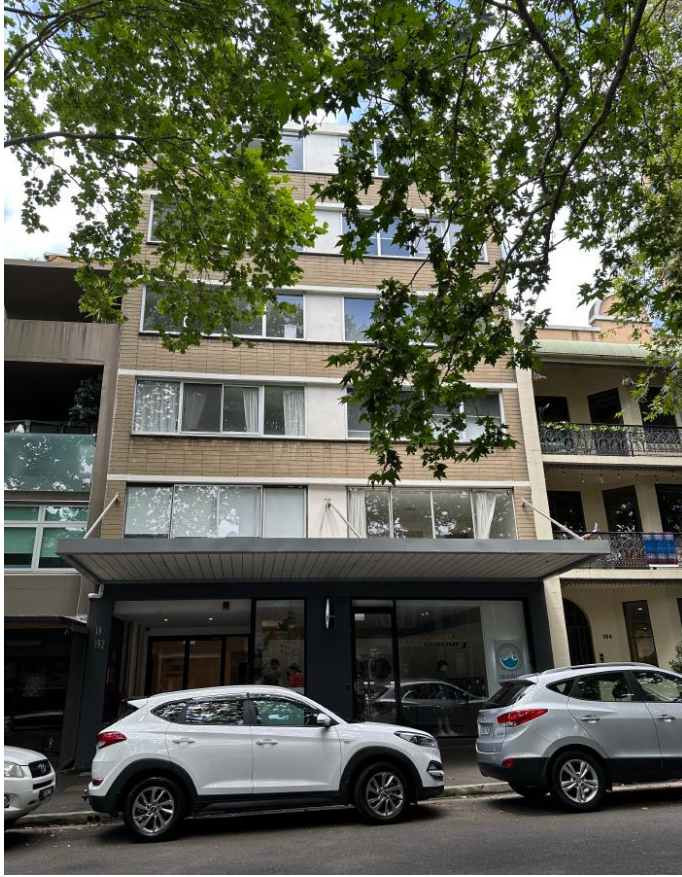
Figure 2: Site viewed from Victoria Street, looking east.
